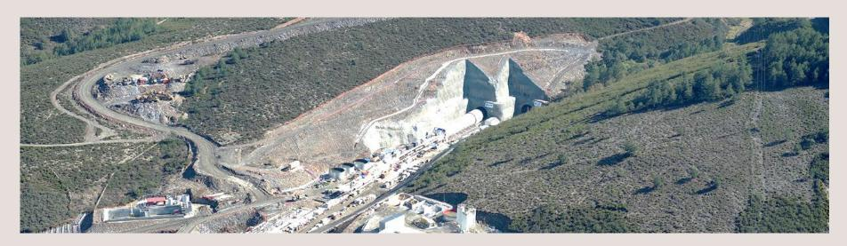
Bolaños tunnel is a 6.8 km twin High Speed Rail tunnel. Each tube has 11 m diameter and is bored by a simple shield TBM. The maximum overburden is about 200 m with a water load of 140 m.
